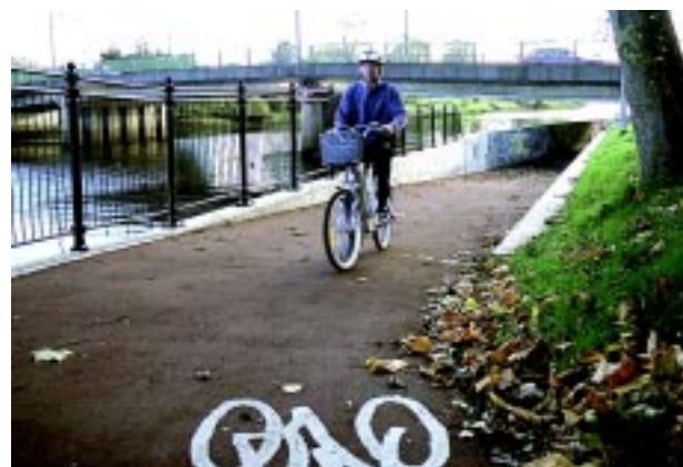
The Governor's Bridge cycle underpass in Belfast, opened in summer 2001, enables pedestrians and cyclists to cross safely under a heavily trafficked bridge and is only the second of its type in Europe.
